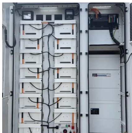
Battery energy storage system (BESS) container. ...
